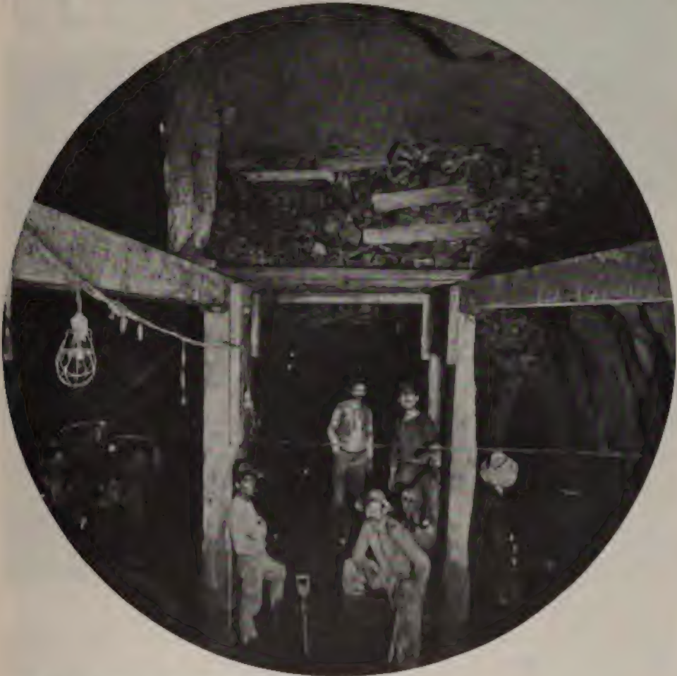
—every • • • precaution known to the engineering art was taken
